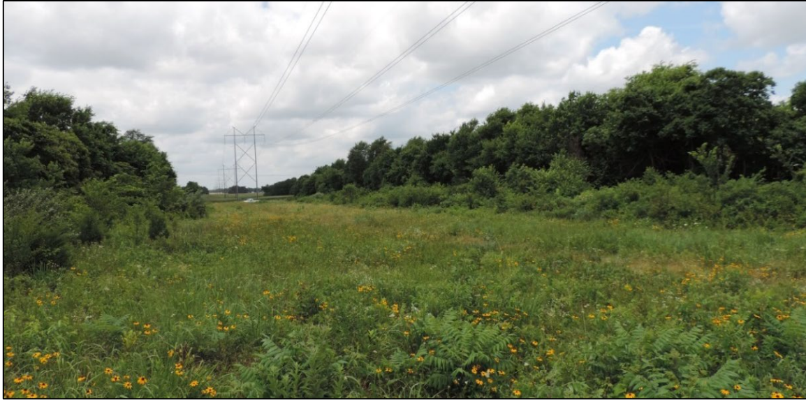
Figure 5 Wire Zone – Border Zone on LU Transmission ROW
