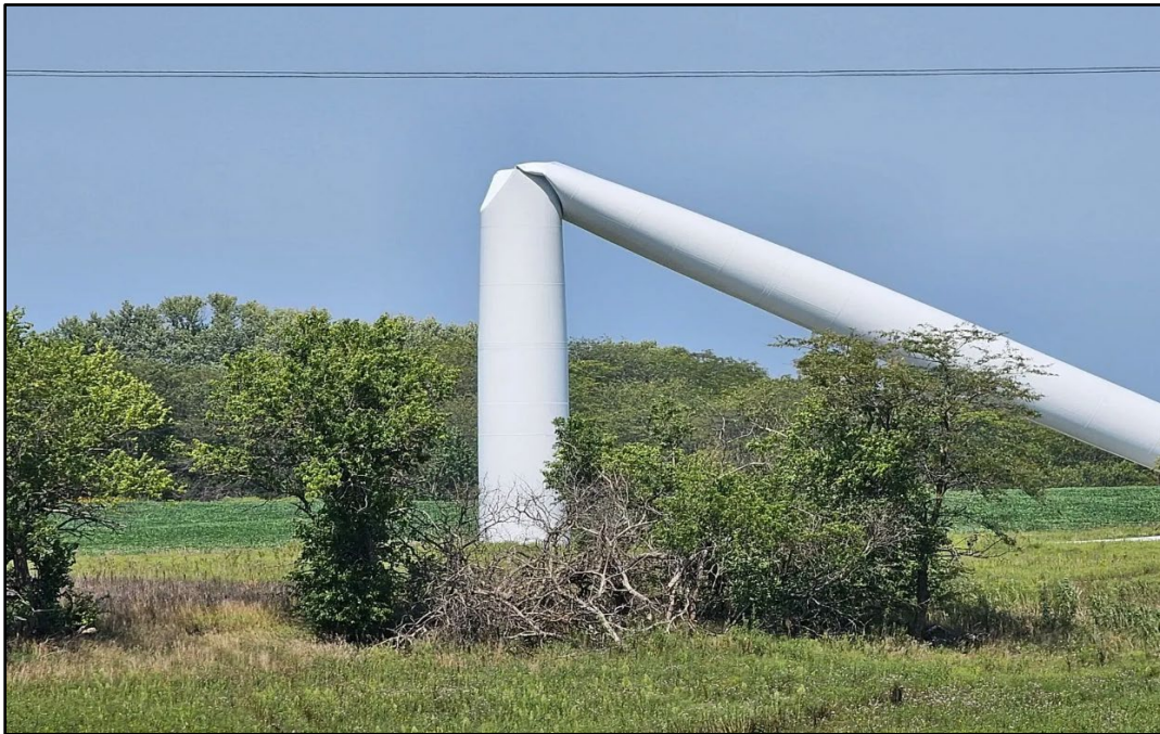
3 Figure 2: High Prairie Renewable Energy Center – 2 nd Wind Turbine to collapse August 25 th , 2024. 3
