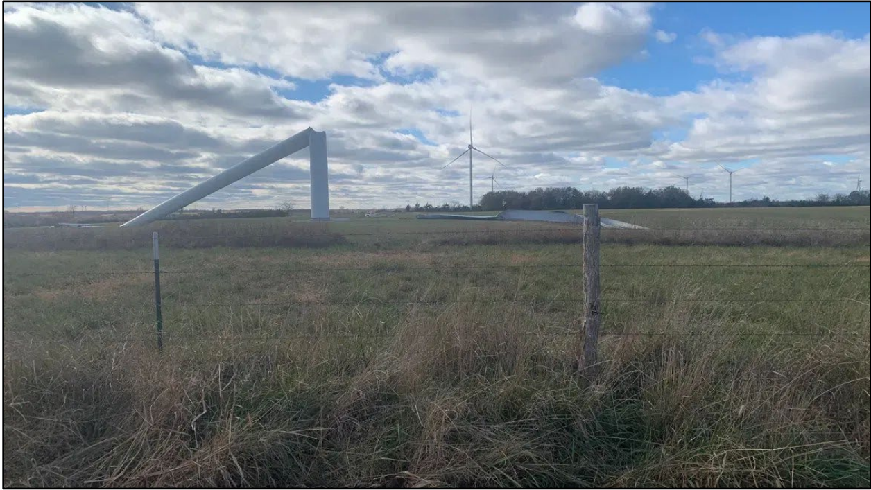
1 Figure 3: High Prairie Renewable Energy Center – 3 rd Wind Turbine to collapse October 31 st , 2024. 4
