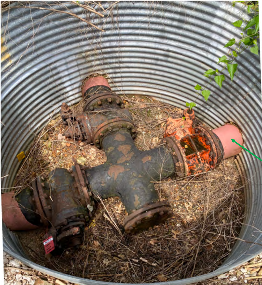
Figure 4: Photograph of the Valve Cluster Pit that contains the cross-tee fitting. Taken by City Utilities Prior to the July 17, 2023 Natural Gas Incident, Springfield Missouri (Source City Utilities of Springfield in response to Staff Data Request 0006)
