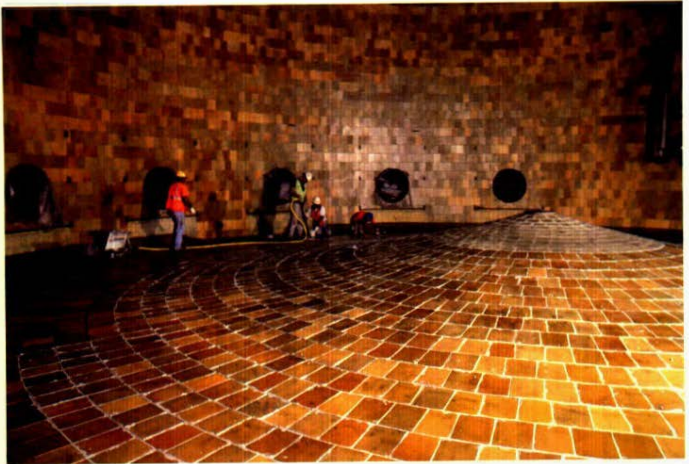
Inside of Unit 1 Absorber During Stebbins Tile Installation
