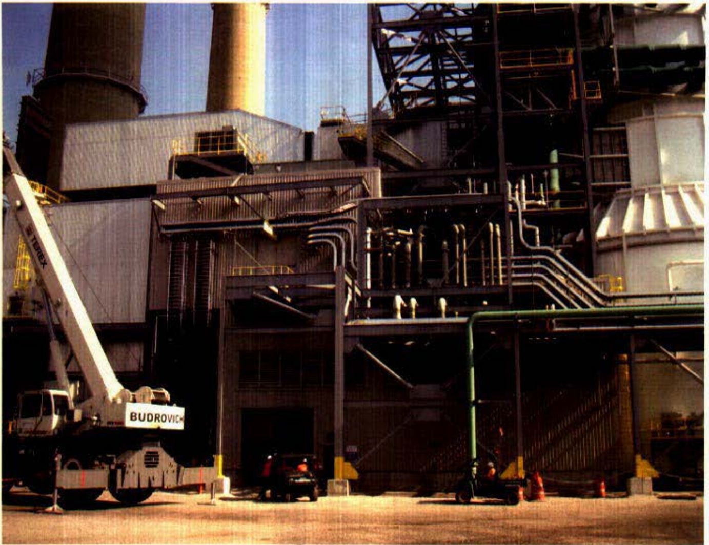
New Absorber Building As Seen From Unit 2 Side
