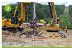
3 Dig structure holes
