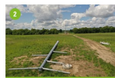
2 Assemble structure on the ground
