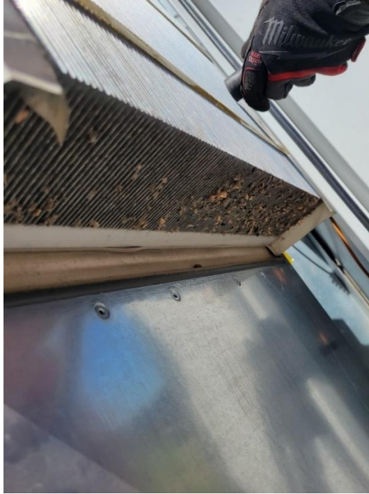
Inverter module heat sink cleaning
