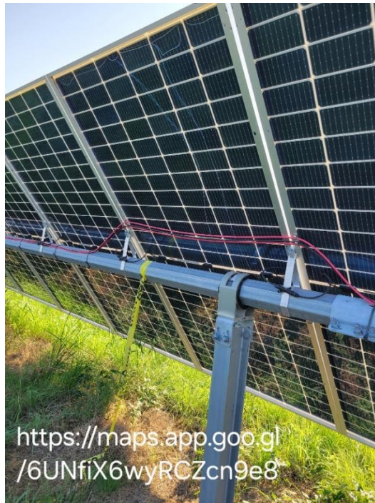
Cracked solar panel (rear glass)
