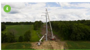
4 Lift structure into hole and backfill with concrete
