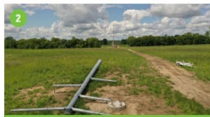
2 Assemble structure on the ground
