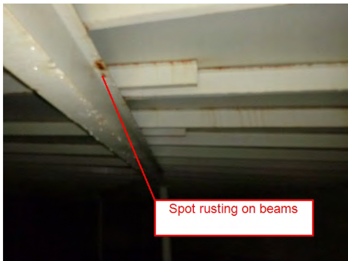
Rust streaking from top of beams
