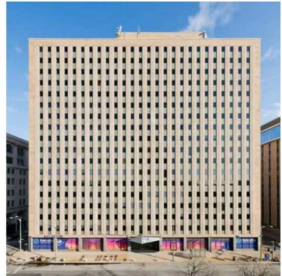
Example Data Center on Tucker, Downtown
