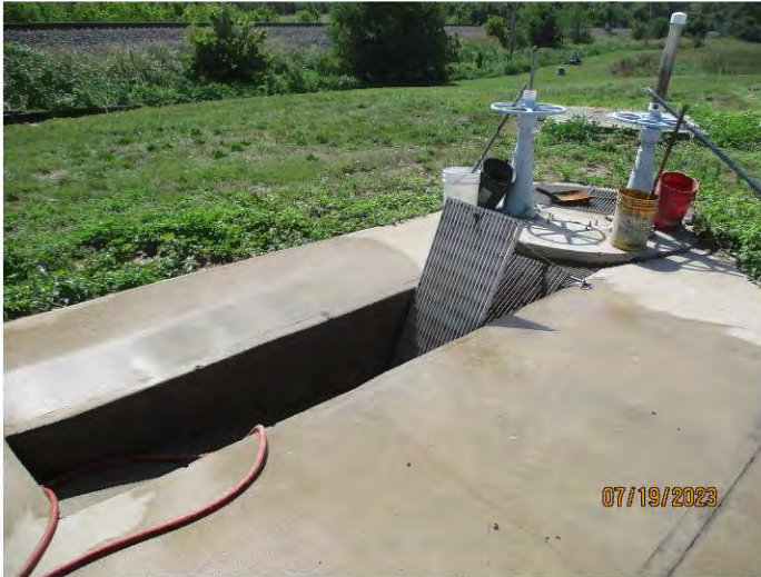
Photo #: 1 Taken by: Joshua Grosvenor Entity: Neosho WWTP Permit: MO0104906 Location: Neosho Shoal Creek Description: Receiving station for hauled wastewater. Date Taken: July 19, 2023 Media: WPCB
