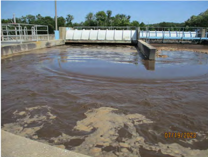
Photo #: 4 Taken by: Joshua Grosvenor Entity: Neosho WWTP Permit: MO0104906 Location: Neosho Shoal Creek Description: Oxidation Ditch Date Taken: July 19, 2023 Media: WPCB
