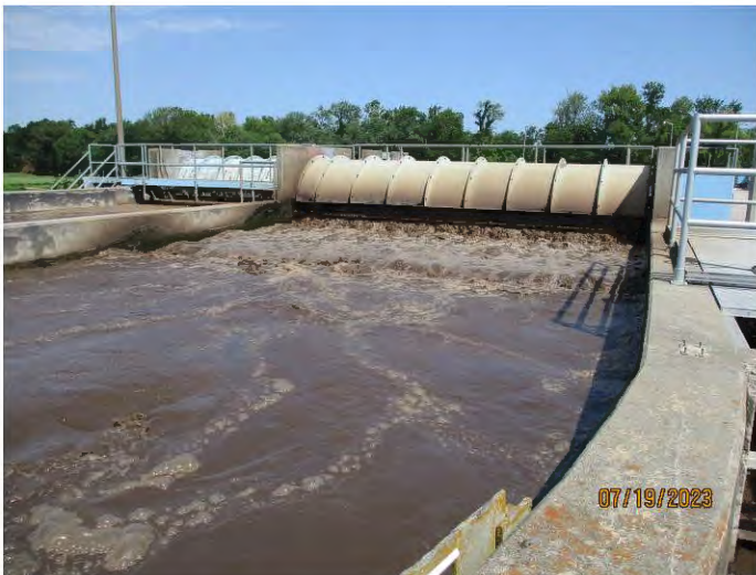
Photo #: 5 Taken by: Joshua Grosvenor Entity: Neosho WWTP Permit: MO0104906 Location: Neosho Shoal Creek Description: Oxidation ditch, rotors providing aeration. Date Taken: July 19, 2023 Media: WPCB
