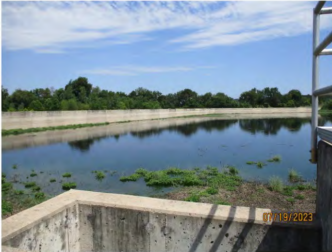
Photo #: 16 Taken by: Joshua Grosvenor Entity: Neosho WWTP Permit: MO0104906 Location: Peak flow basin Description: Peak flow basin, eight million gallons. Date Taken: July 19, 2023 Media: WPCB
