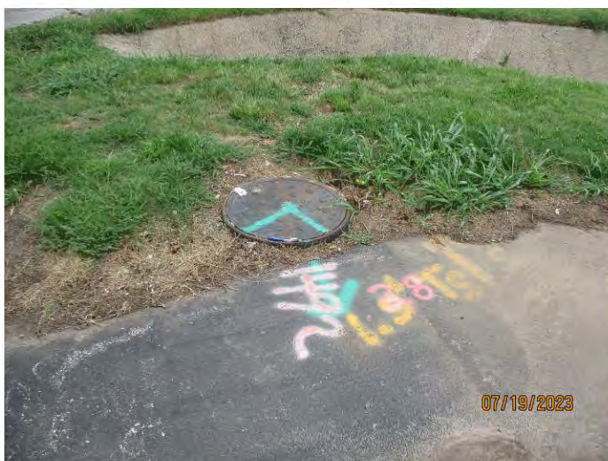
Photo #: 27 Taken by: Joshua Grosvenor Entity: Neosho WWTP Permit: MO0104906 Location: S Neosho Boulevard and W South Street Description: Manhole with the greatest frequency of overflows, during high flow events. Date Taken: July 19, 2023 Media: WPCB
