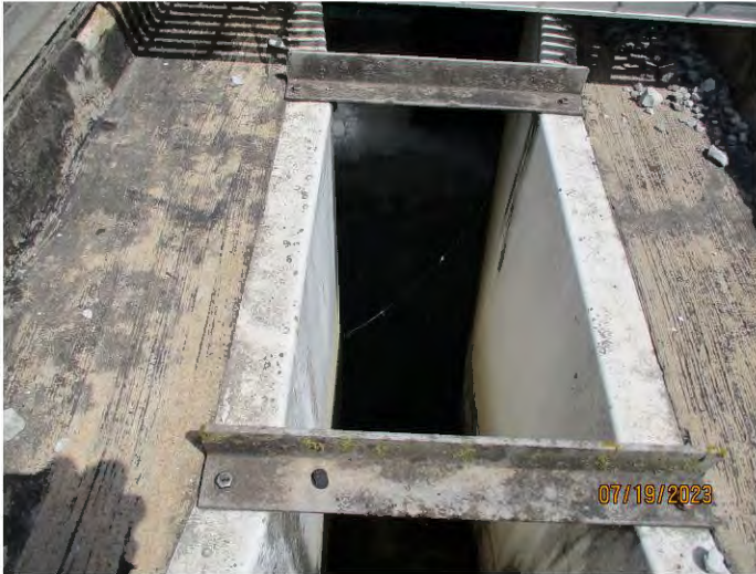
Photo #: 10 Taken by: Joshua Grosvenor Entity: Neosho WWTP Permit: MO0104906 Location: Neosho Shoal Creek Description: Parshall flume flow measurement. Date Taken: July 19, 2023 Media: WPCB
