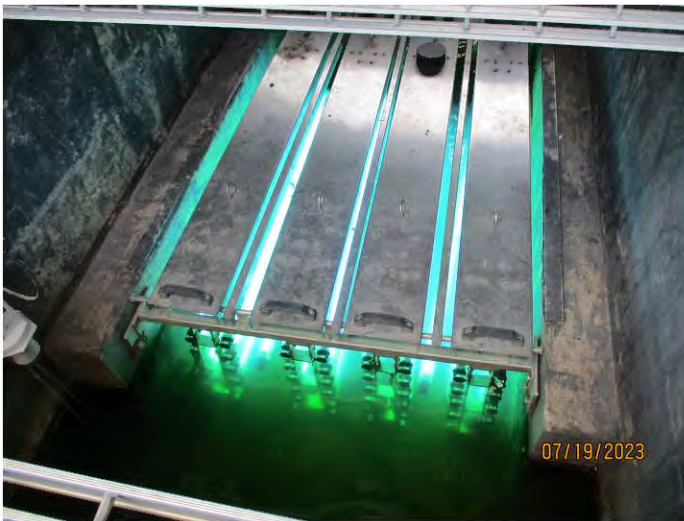
Photo #: 11 Taken by: Joshua Grosvenor Entity: Neosho WWTP Permit: MO0104906 Location: Neosho Shoal Creek Description: Ultraviolet disinfection unit, functioning. Date Taken: July 19, 2023 Media: WPCB
