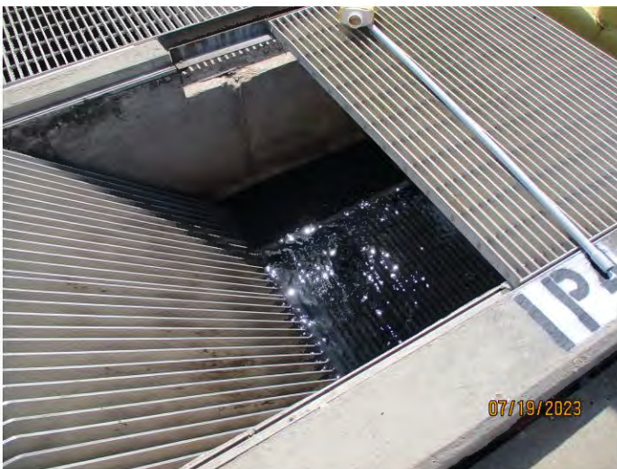
Photo #: 3 Taken by: Joshua Grosvenor Entity: Neosho WWTP Permit: MO0104906 Location: Neosho Shoal Creek Description: Bar screen. Date Taken: July 19, 2023 Media: WPCB
