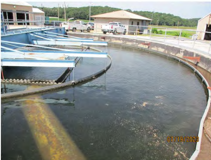
Photo #: 6 Taken by: Joshua Grosvenor Entity: Neosho WWTP Permit: MO0104906 Location: Neosho Shoal Creek Description: Operational clarifier. Date Taken: July 19, 2023 Media: WPCB
