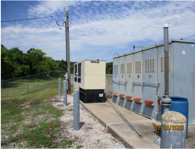
Photo #: 19 Taken by: Joshua Grosvenor Entity: Neosho WWTP Permit: MO0104906 Location: Peak flow basin Description: Peak flow basin backup generators, exercised regularly. Date Taken: July 19, 2023 Media: WPCB
