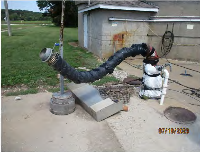
Photo #: 13 Taken by: Joshua Grosvenor Entity: Neosho WWTP Permit: MO0104906 Location: Neosho Shoal Creek Description: Hook up for sludge hauling trucks to load sludge. Date Taken: July 19, 2023 Media: WPCB
