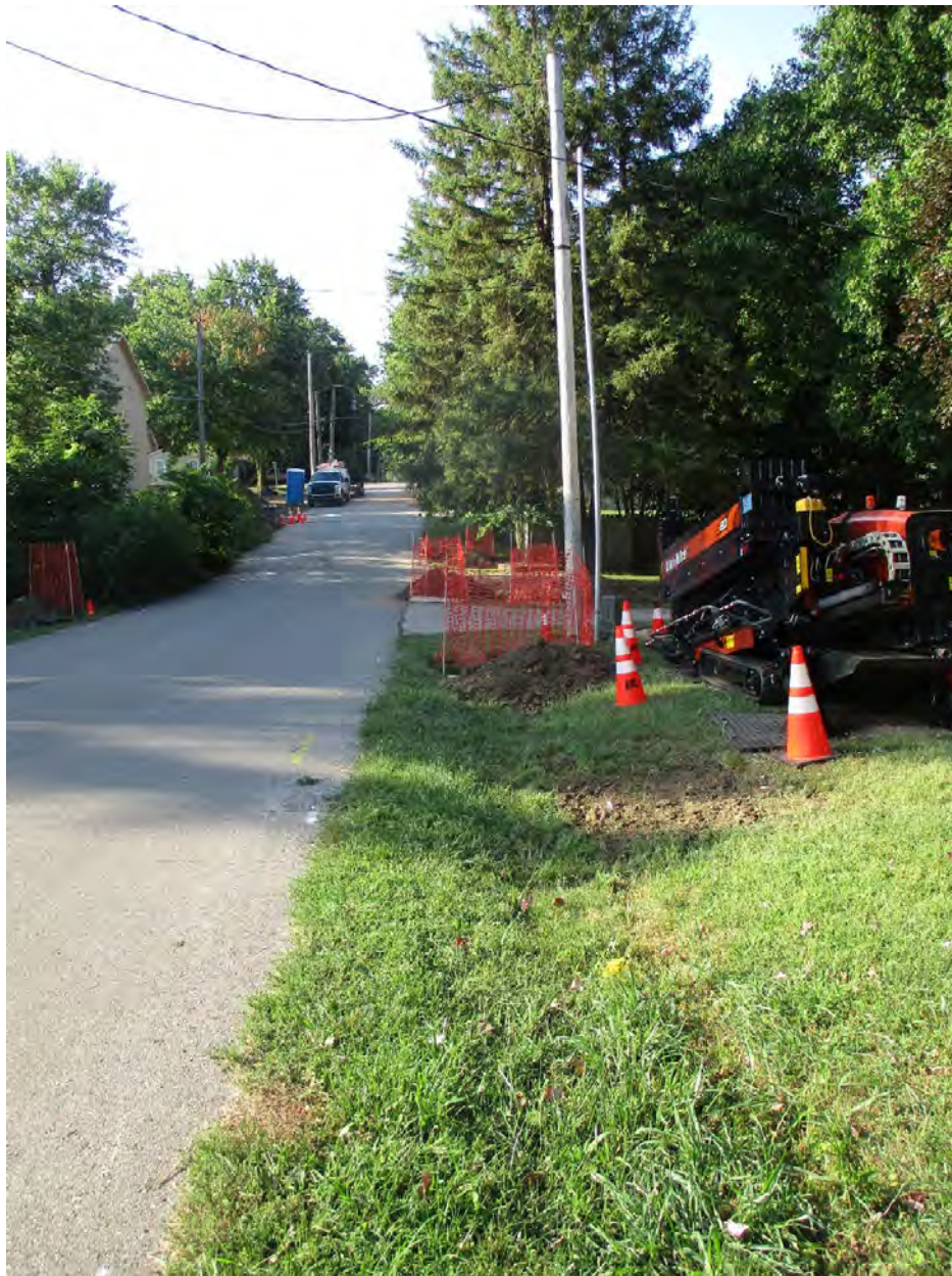
Figure 4 – Photograph looking south along South Hocker Ave. The horizontal directional drilling machine is set up on right side of image in order to install telecommunications line heading south alongside South Hocker Ave. (Staff photograph)
