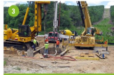
3 Dig structure holes
