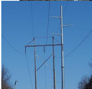
Replacing aged wood structures with steel poles
