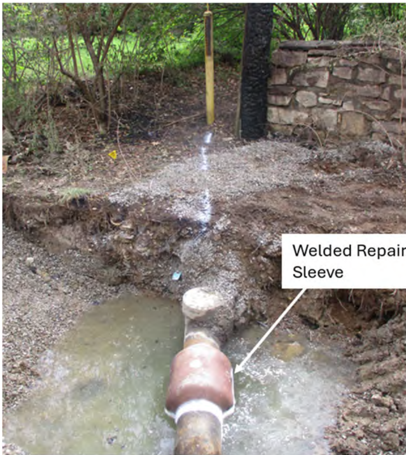
Figure 2: Pipeline Following Repair (Source: Staff Photograph)
