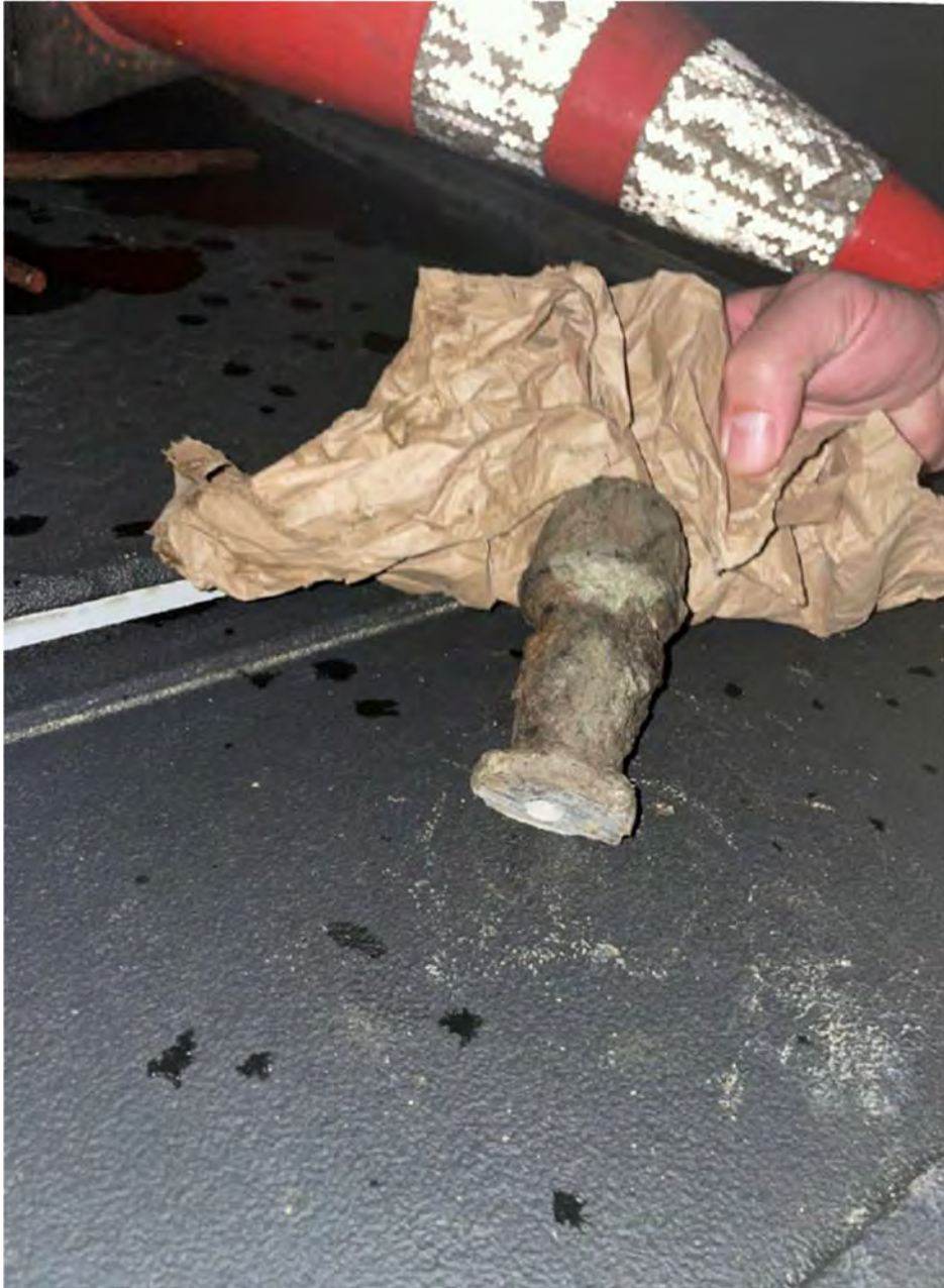
Figure 3: Damaged Fitting After Removal (Source: Spire Response to Staff Data Request 0001.3B)
