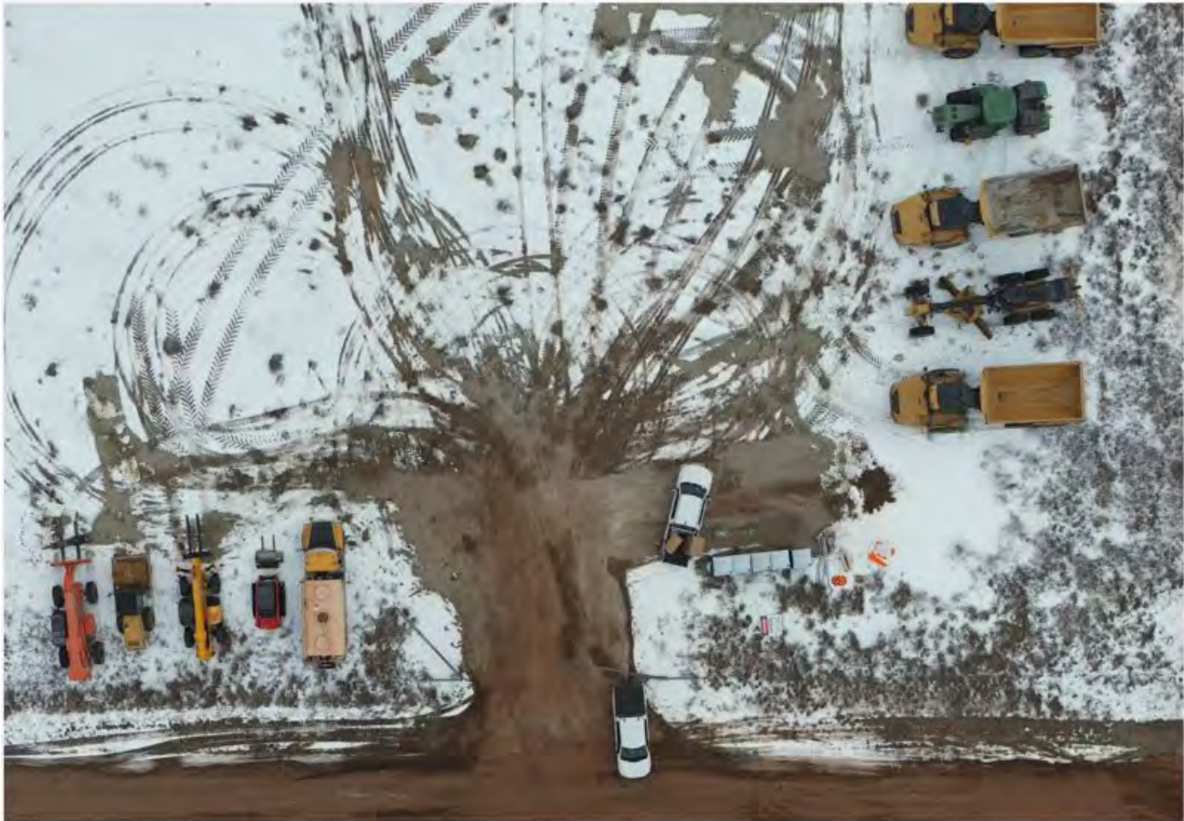
February 2026 – Aerial view of site, prepping for Mobilization
