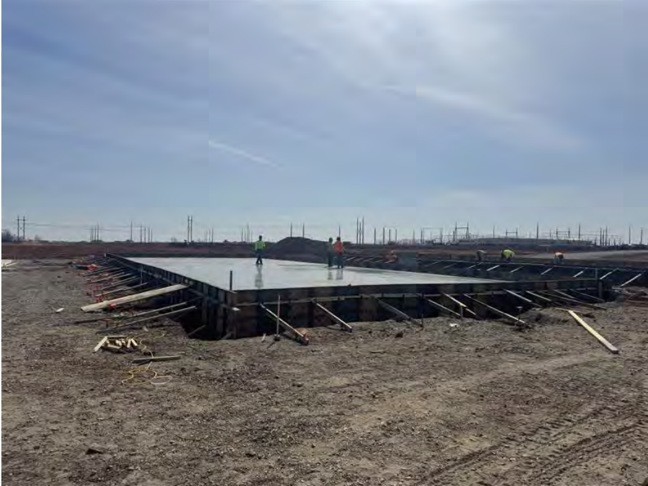
March 2026 – Placement of temporary warehouse concrete
