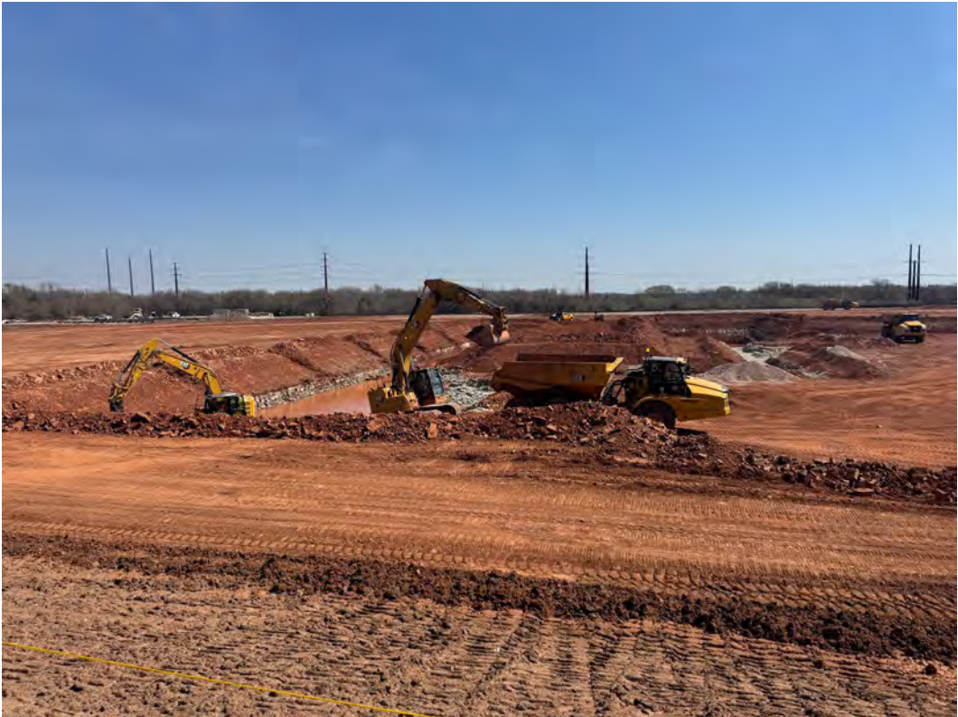
Excavation in Bower Block for duct bank
