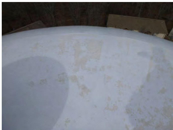
Peeling paint on bowl roof
