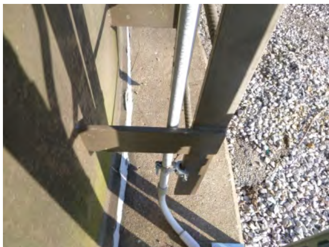
Sealant damaged at lower flange
