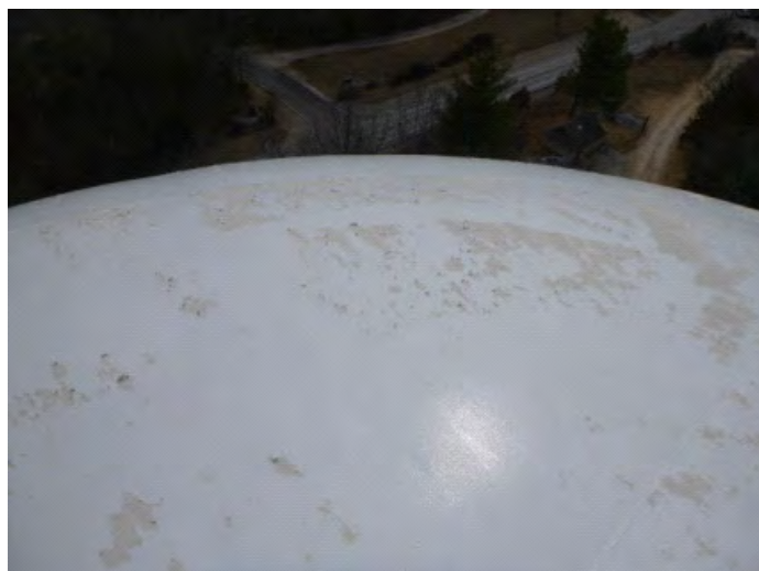
Peeling paint on bowl roof
