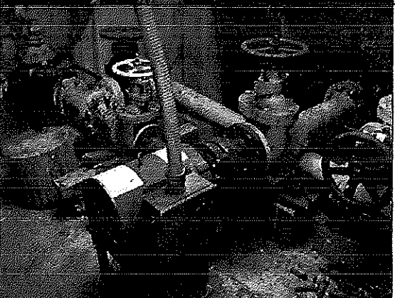
Photo #:8 Date Taken: 08/20/2014 By: Michelle Oglesby Program: PDWB File: Crawford County Location: Indian Hills Utilities Description: Pump and piping within the well house for Well #1.
