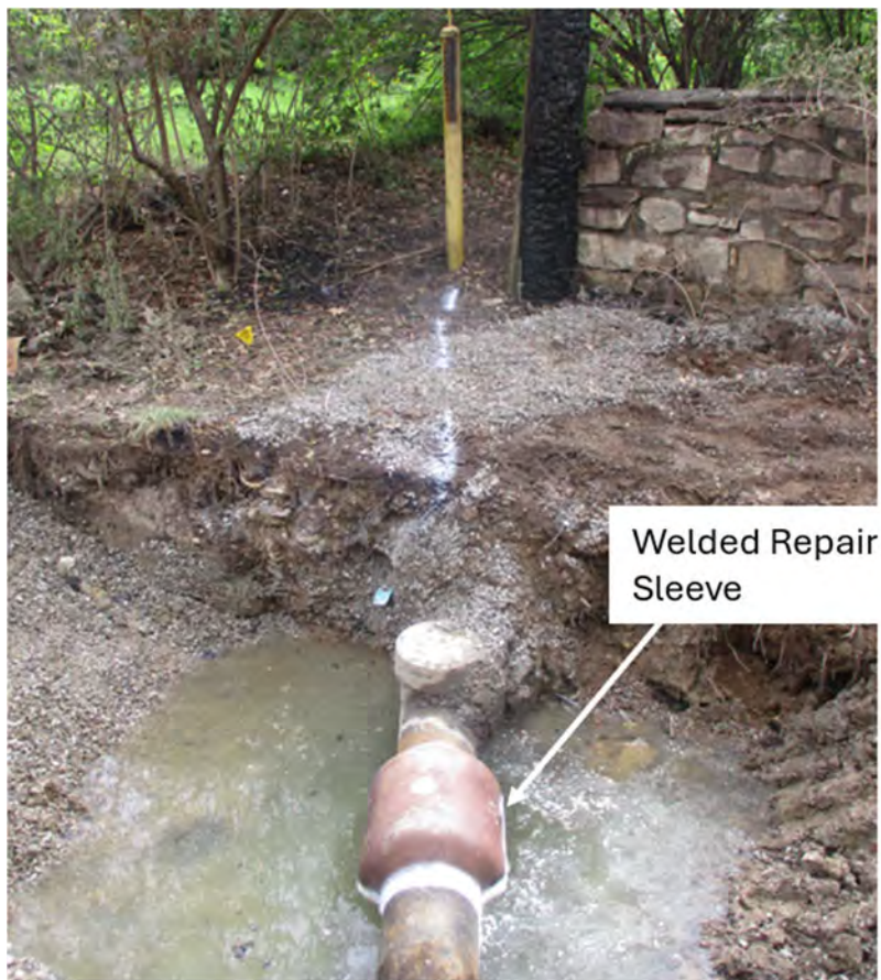
Figure 2: Pipeline Following Repair (Source: Staff Photograph)
