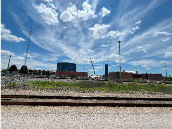
Photo 1 Taken By: Christina Kerr Entity: Blue River Wastewater Treatment Plant Facility ID: 095-0039 Location: 7300 Hawthorne Road, Kansas City Description: Overview of facility. Date Taken: July 2, 2025 Media: Air Pollution Control
