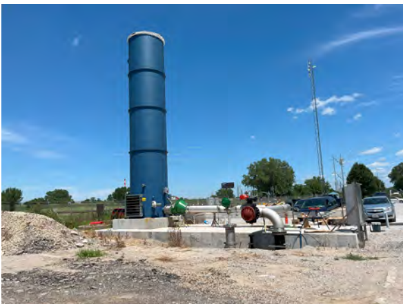
Photo 9 Taken By: Christina Kerr Entity: Blue River Wastewater Treatment Plant Facility ID: 095-0039 Location: 7300 Hawthorne Road, Kansas City Description: New flare that is currently under construction. Date Taken: July 2, 2025 Media: Air Pollution Control
