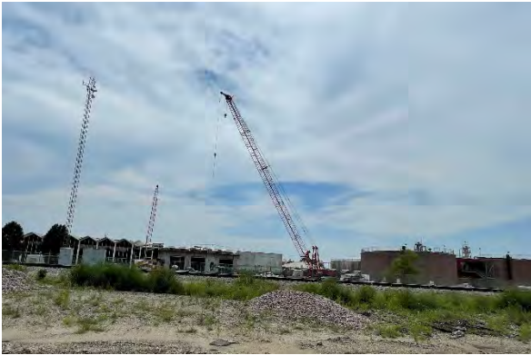
Photo #: 1 Taken By: Christina Kerr Entity: Blue River WWTP Permit: 095-0039 Location: 7300 Hawthorne Road, Kansas City Description: Facility overview from the north. Date Taken: July 25, 2023 Media: KCRO Air Unit
