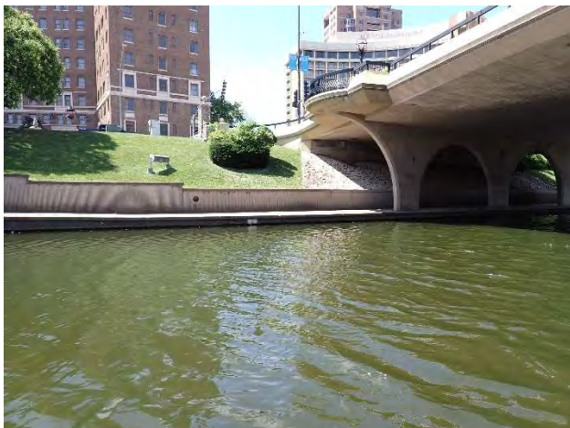
Photo: 24 Taken By: Denise Eagan Entity: Kansas City Permit: MO0024911 Location: 39.040482, -94.591234 Description: Viewing permitted feature Combined Sewer Outfall 014 Date Taken: June 10, 2025 Media: CW
