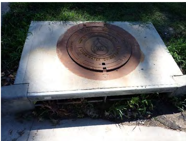
Photo: 3 Taken By: Denise Eagan Entity: Kansas City Permit: MO0024911 Location: 39.051207, -94.537651 Description: Viewing the newly installed storm sewer at Monroe Ave. Date Taken: June 10, 2025 Media: CW
