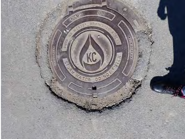
Photo: 1 Taken By: Denise Eagan Entity: Kansas City Permit: MO0024911 Location: 39.053480, -94.541017 Description: Viewing the new manhole cover on the newly separated sanitary sewer on Monroe Ave. Date Taken: June 10, 2025 Media: CW
