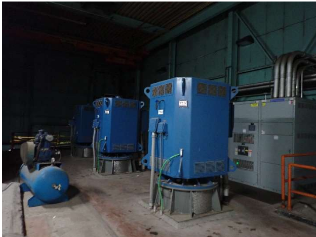
Photo: 8 Taken By: Denise Eagan Entity: Kansas City Permit: MO0024911 Location: 39.085257, -94.606802 Description: Viewing the pump motors of the Turkey Creek Pump Station. Date Taken: June 10, 2025 Media: CW
