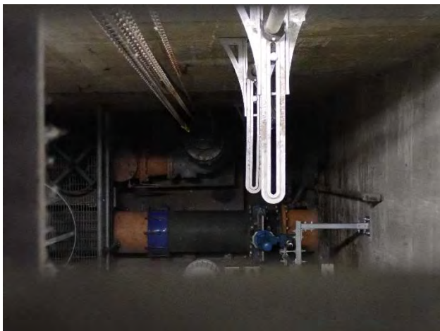
Photo: 12 Taken By: Denise Eagan Entity: Kansas City Permit: MO0024911 Location: 39.076999, -94.602132 Description: Viewing the sanitary sewer (top) and stormwater line (bottom). Date Taken: June 10, 2025 Media: CW
