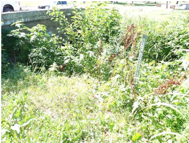
Photo: 23 Taken By: Denise Eagan Entity: Kansas City Permit: MO0024911 Location: 7300 Hawthorne Rd Description: Viewing the outfall for diversion structure 113 with the sign missing. Date Taken: June 10, 2025 Media: CW
