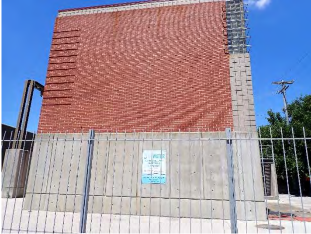
Photo: 10 Taken By: Denise Eagan Entity: Kansas City Permit: MO0024911 Location: 39.076999, -94.602132 Description: Viewing the Southeast Blvd flood pumping station. Date Taken: June 10, 2025 Media: CW
