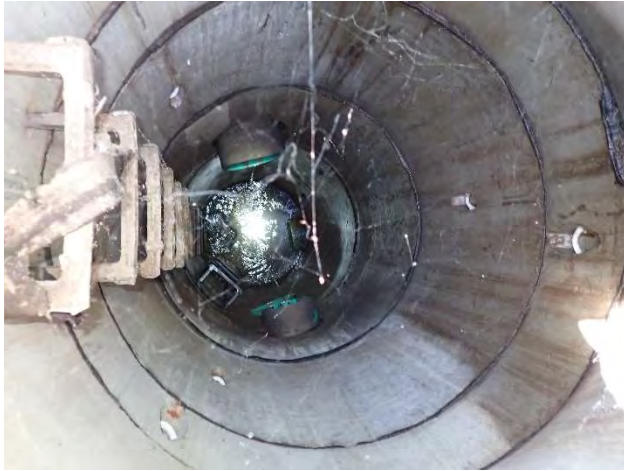
Photo: 4 Taken By: Denise Eagan Entity: Kansas City Permit: MO0024911 Location: 39.050970, -94.534135 Description: Viewing the new manhole on Spruce which has the diversion structure removed. Date Taken: June 10, 2025 Media: CW
