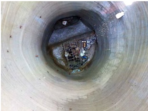
Photo: 18 Taken By: Denise Eagan Entity: Kansas City Permit: MO0024911 Location: 39.006741, -94.569577 Description: Viewing inside CSO Permitted Feature 097 diversion with overflow grate visible. Date Taken: June 10, 2025 Media: CW
