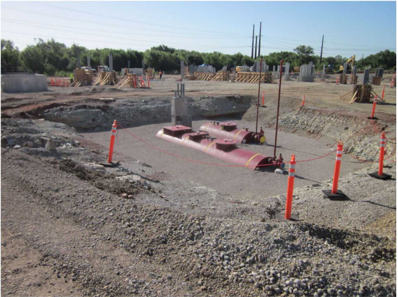
June 2026 - Installed and backfilled oil water separator
