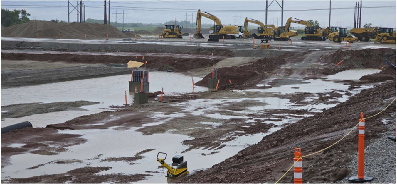
May 2026 – Conditions on site during heavy rain fall
