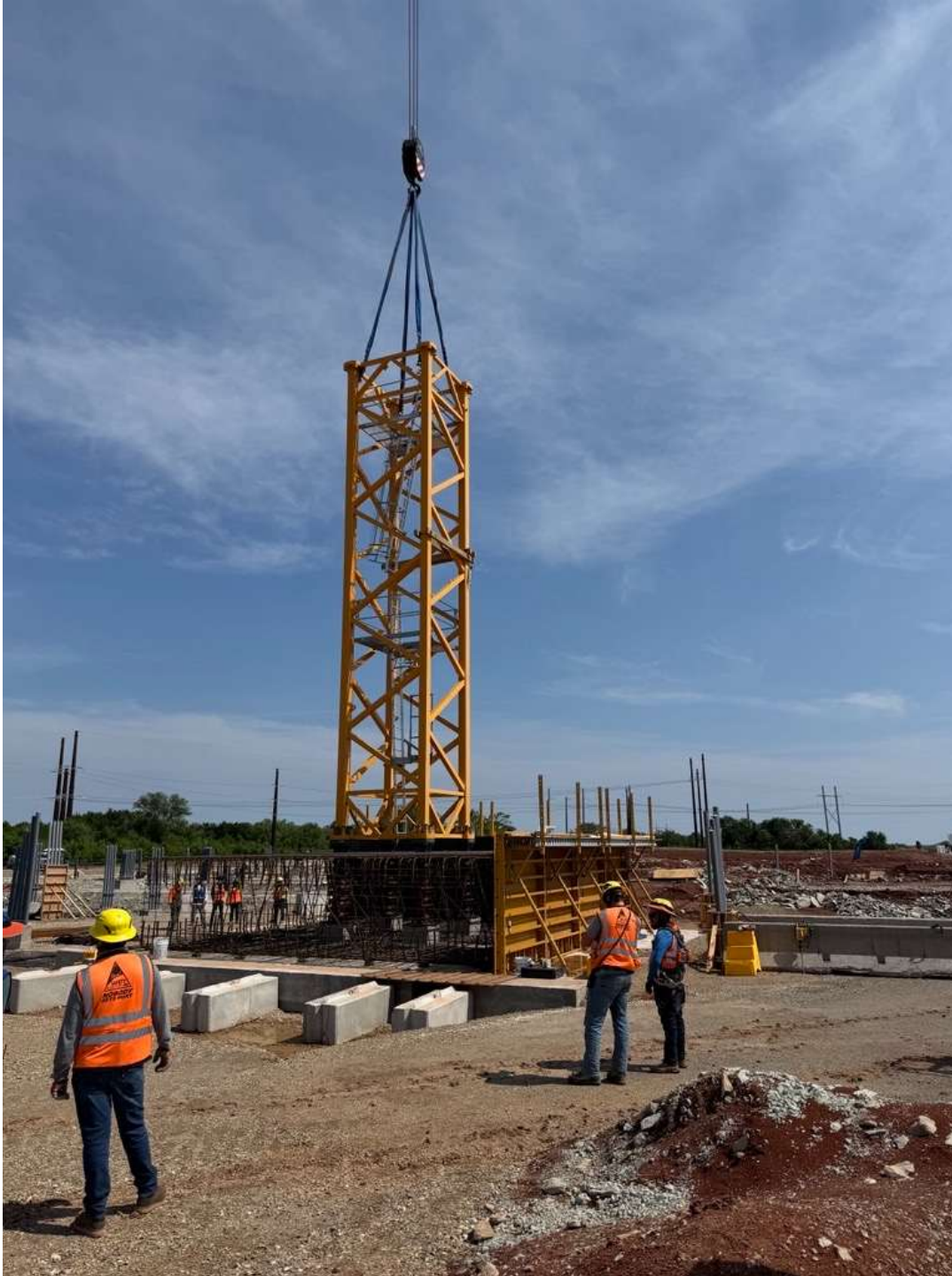
June 2026 - Tower crane assembly
