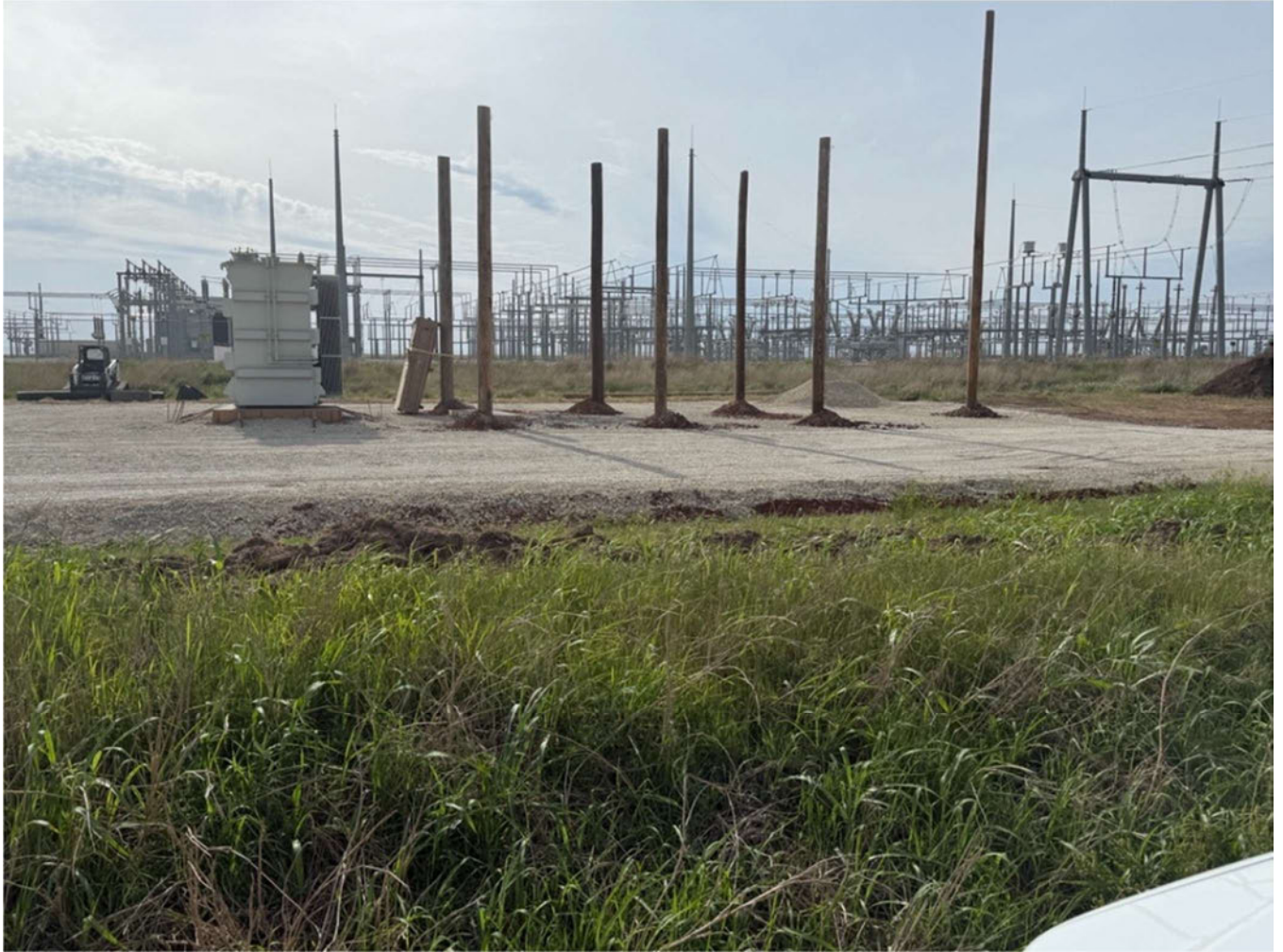
May 2026 - Transformer set on temporary substation
