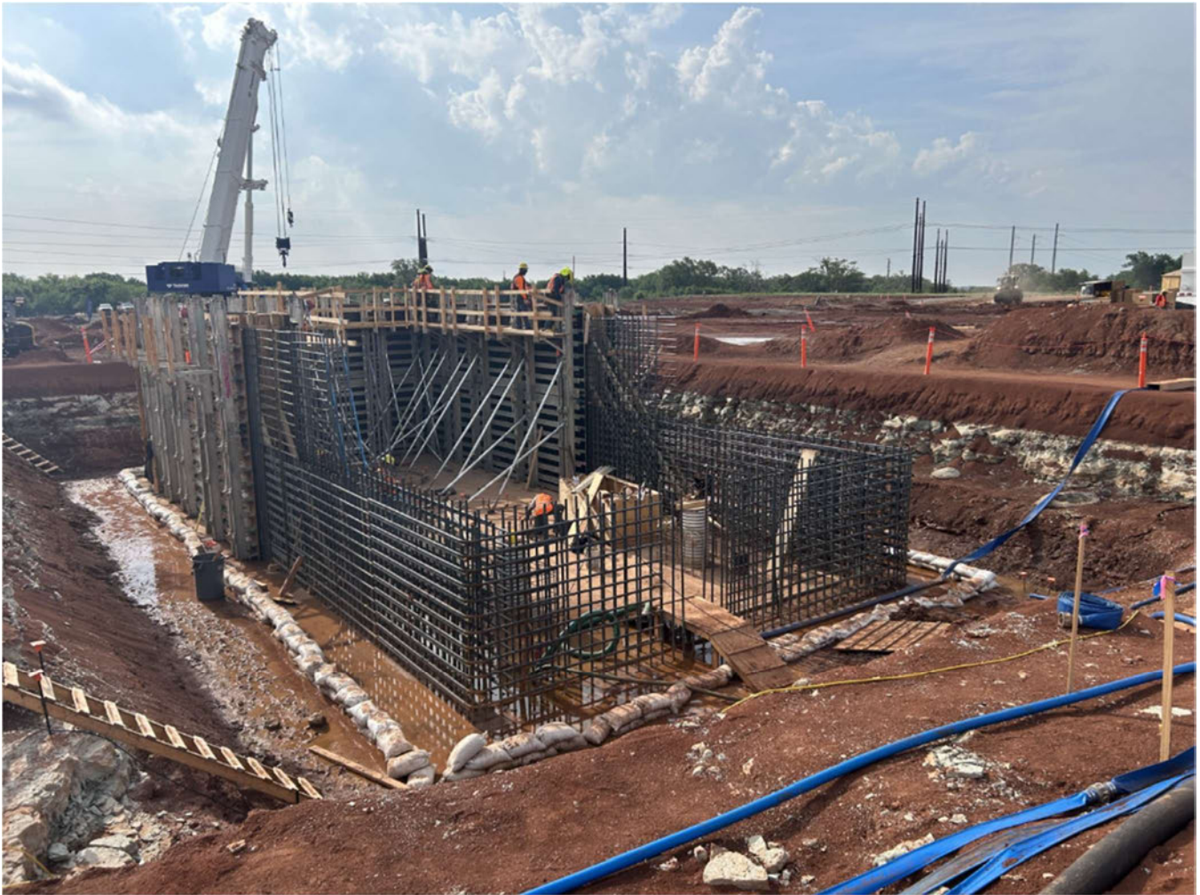
June 2026 - ST drains pit tank wall concrete form installation
