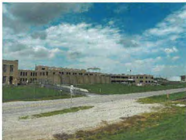
VIEW OF FILTRATION PLANT
