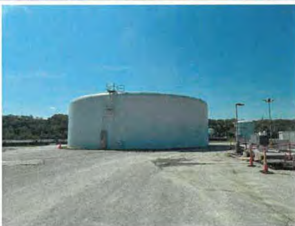
VIEW OF STORAGE TANK
