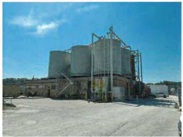
VIEW OF CHEMICAL PLANT
