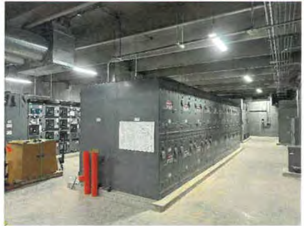
HIGH SERVICE BUILDING
