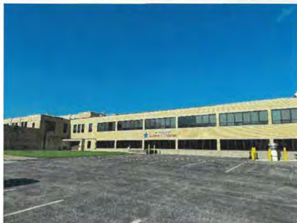
VIEW OF FILTRATION PLANT
