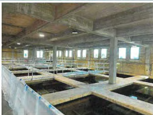
VIEW OF FILTRATION PLANT
