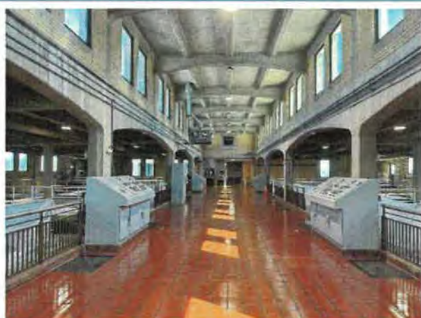
VIEW OF FILTRATION PLANT
