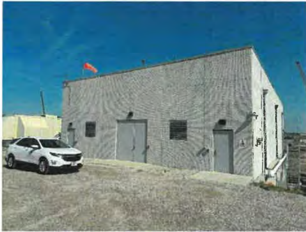
HIGH SERVICE BUILDING
