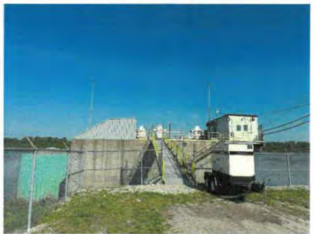
INTAKE PUMP HOUSE
