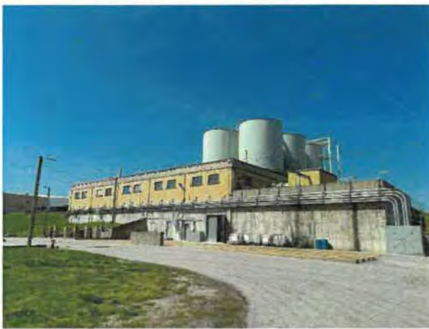
VIEW OF CHEMICAL PLANT
