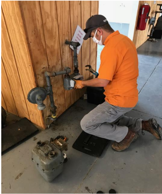
Training – How to install a Smart Meter MO West
