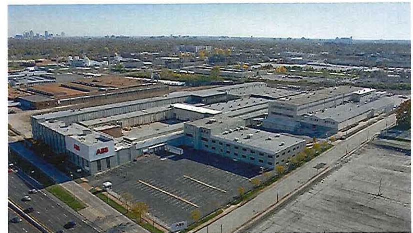
ABB’s manufacturing and repair facility in St. Louis.
