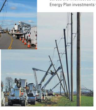
A new sub-transmission line was directly hit by the tornado. The line was installed in 2020 specifically to protect customers from storms and high winds. The composite poles prevented a cascading collapse and failure. While damage did occur, the composite poles were found to be undamaged and only needed to be straightened. Power was restored in half the time thanks to these new upgrades.
