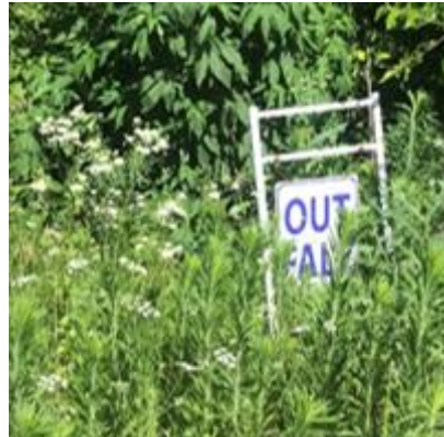
Outfall inaccessible at Country Hill Estates due to vegetation overgrowth.
