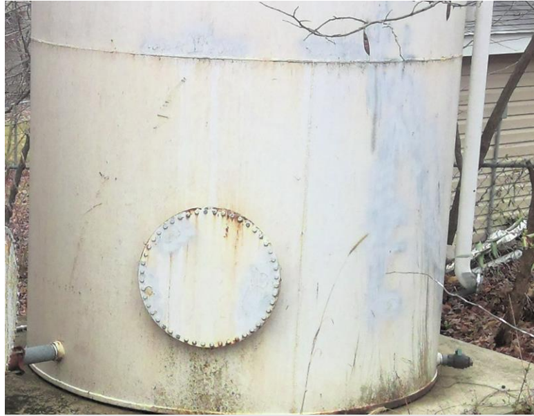
Point repairs on ground storage tank (note slightly different paint color)
