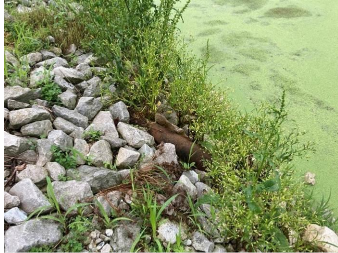
Typical condition of berms and duckweed layer on lagoon surface
