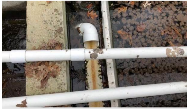
Poor condition of clarifier at Chelsea Rose
