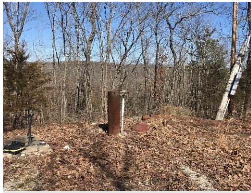
Well #2 – note rusting and lack of fencing
