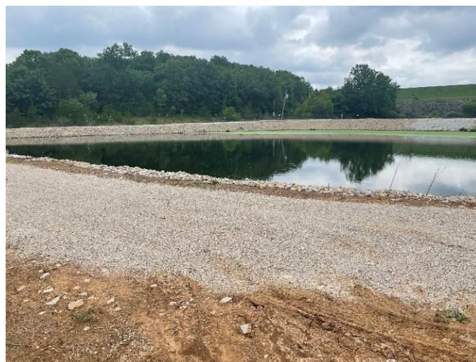
Berms following repairs and application of rip rap
