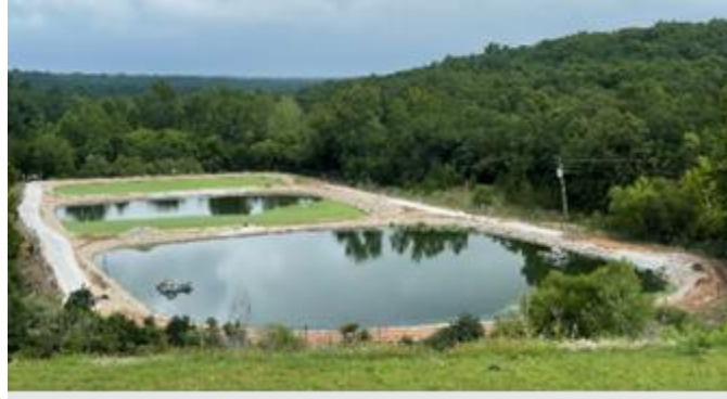
Cleared and rock-lined berms and paths around lagoon
