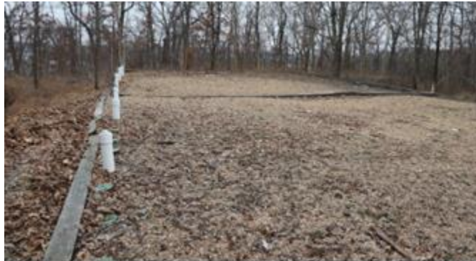
No fencing present at the Cimarron Bay treatment plant
