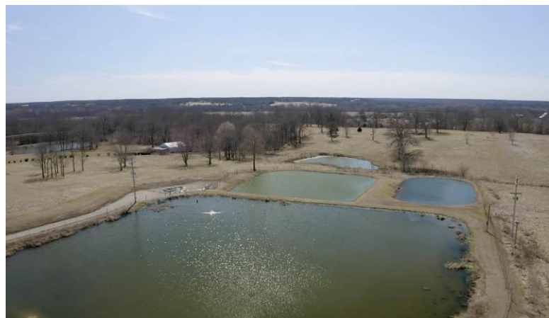
MBBR added to MO Utilities Lagoon
