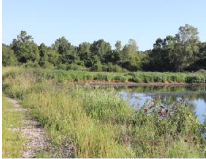
Accumulation of solids in second lagoon and varmint damage to berm visible in background
