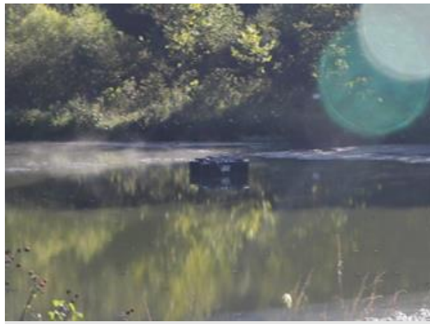
8 9 Failed aerator at Terre du Lac three-cell lagoon 10
