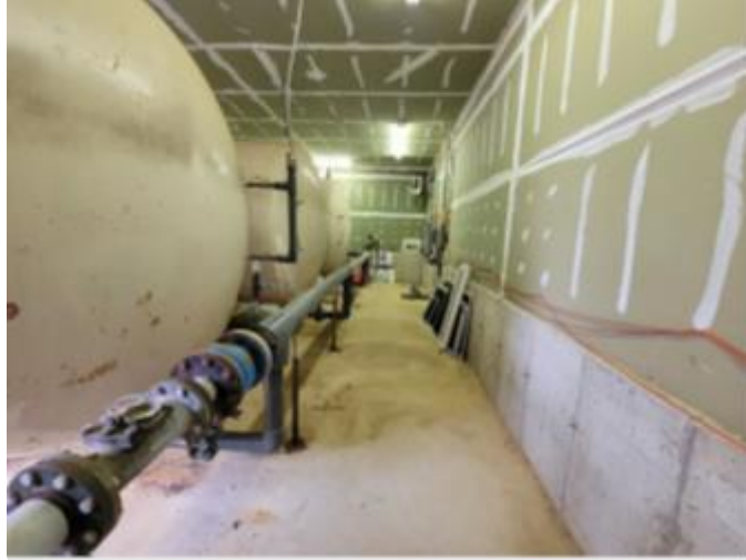
Hydropneumatic storage tank building (note violations associated with dependence on hydropneumatic storage only and use of 2” pvc piping)
