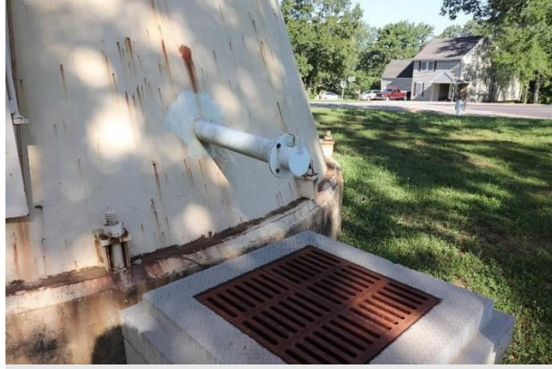
Base of tank near well #4
