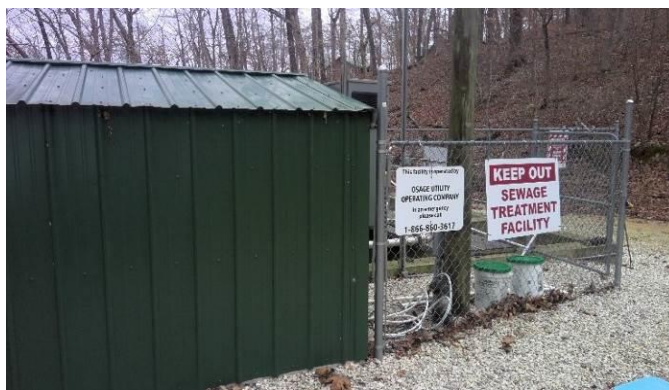
New blower housing and fence area
