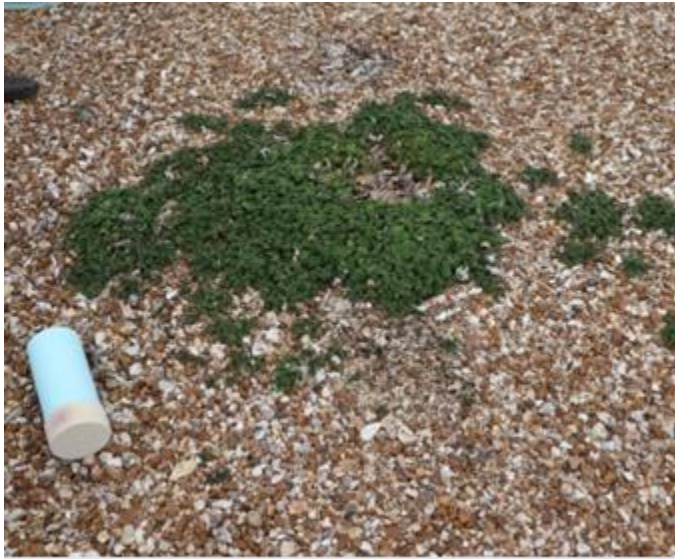
10 11 Vegetation growing on surface of Cedar Glen sand filter
