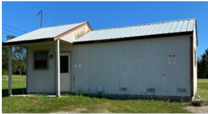
14 15 Well # 3 Well house
