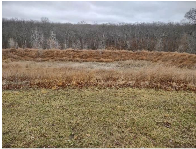
Overgrowth around Missing Well lagoon
