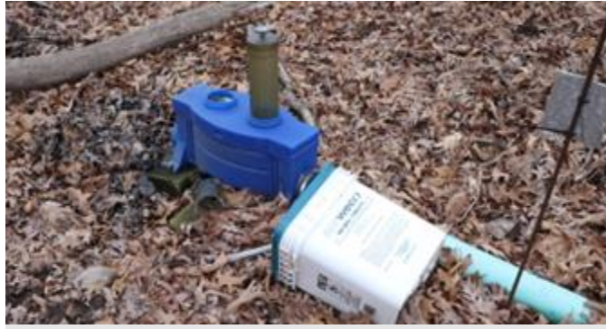
New dechlorination tablet feeder
