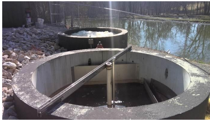
Lake Virginia Lagoon MBBR and clarifier project
