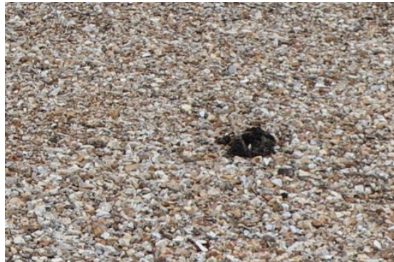
Visible sludge breaking the surface of the Cedar Glen sand filter beds.
