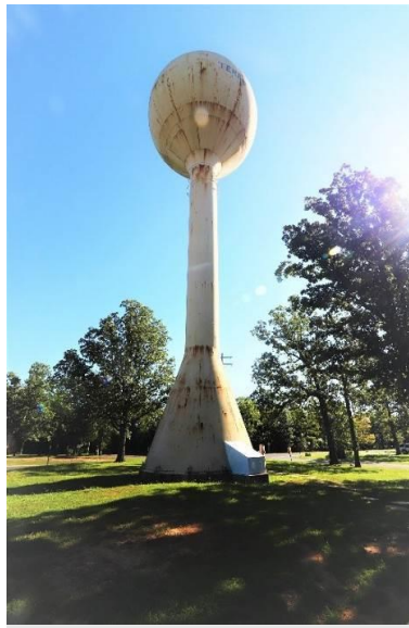
Tank near well #4
