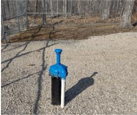
New gravel, well head equipment, and coating at Well #1
