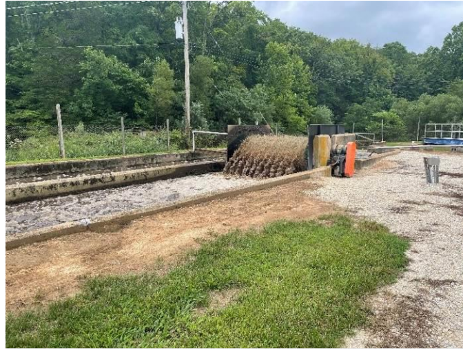
Repaired brush aerator
