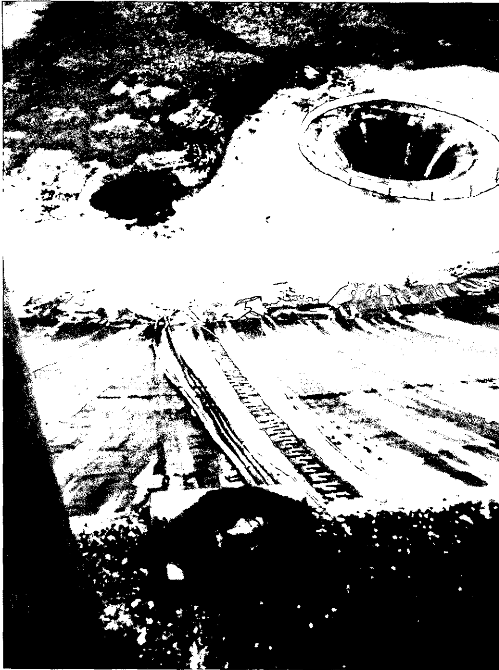
This photograph shows the displacement of the water level measurement sensors (the four black tubes) and the location of the water shaft used for draining and filling the upper reservoir.
