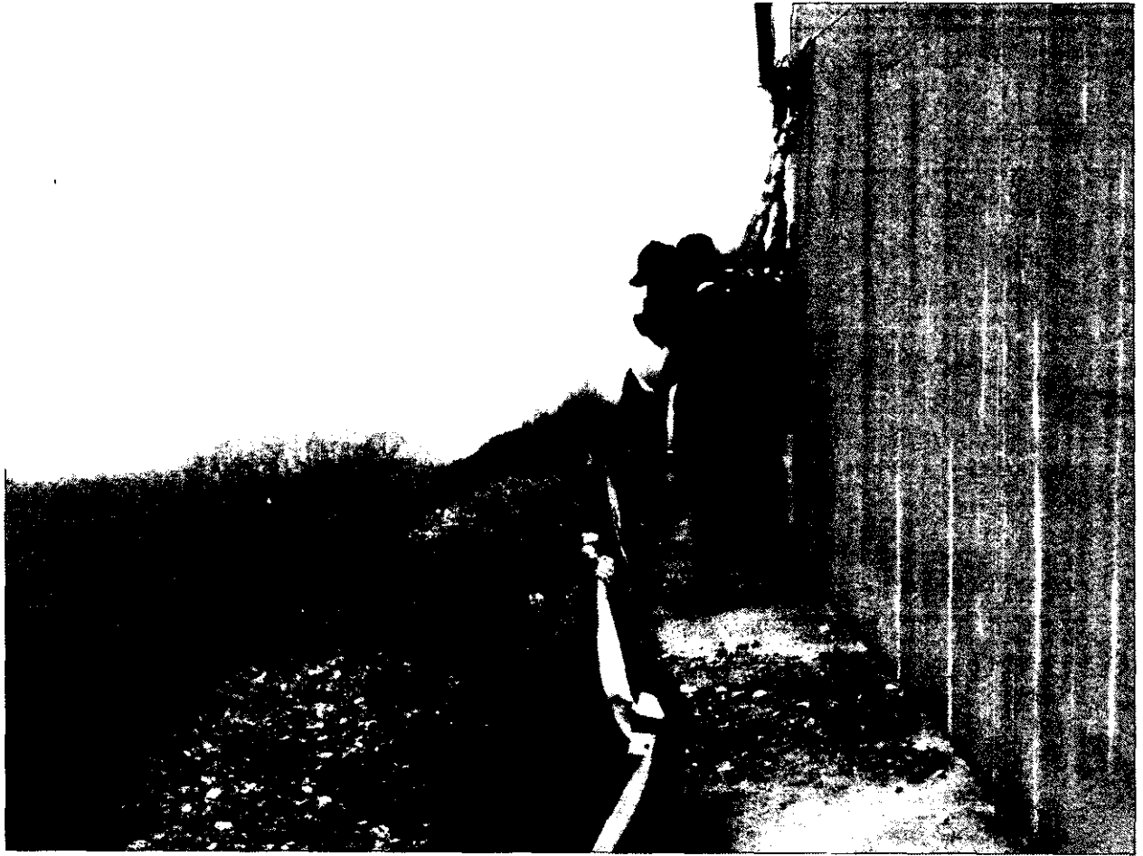
7 8 The photograph above shows a location where the parapet wall was overtopped by water 9 erosion which occurred at several locations around the perimeter of the upper reservoir.
