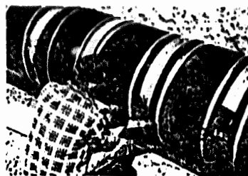
11. Field fabrication: pipes, casings, insulation are assembled at job site
