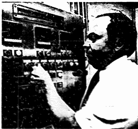
Rich Obremski checks the electrical panel that controls the petrolatum system. Steam is used to melt the petrolatum material used in several Norcliff-Thayer products.
