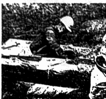
17. Direct-buried pipe ranges in size from 12 to 36 in. for chilled water
