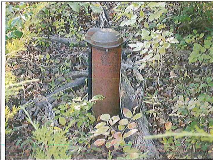
PHOTOGRAPH# 4 TAKEN BY: Darrell Barber ENTITY: Reflections Condos PERMIT: MO3071337 LOCATION: Southeast of well house DESCRIPTION: Abandoned well approximately 135 feet from the public water system well for Reflections Condos. The abandoned well is not located on property owned by Great Southern Bank or Reflections Condominium Owners Association, Inc. DATE TAKEN: August 9, 2017 PROGRAM: Public Drinking Water Branch
