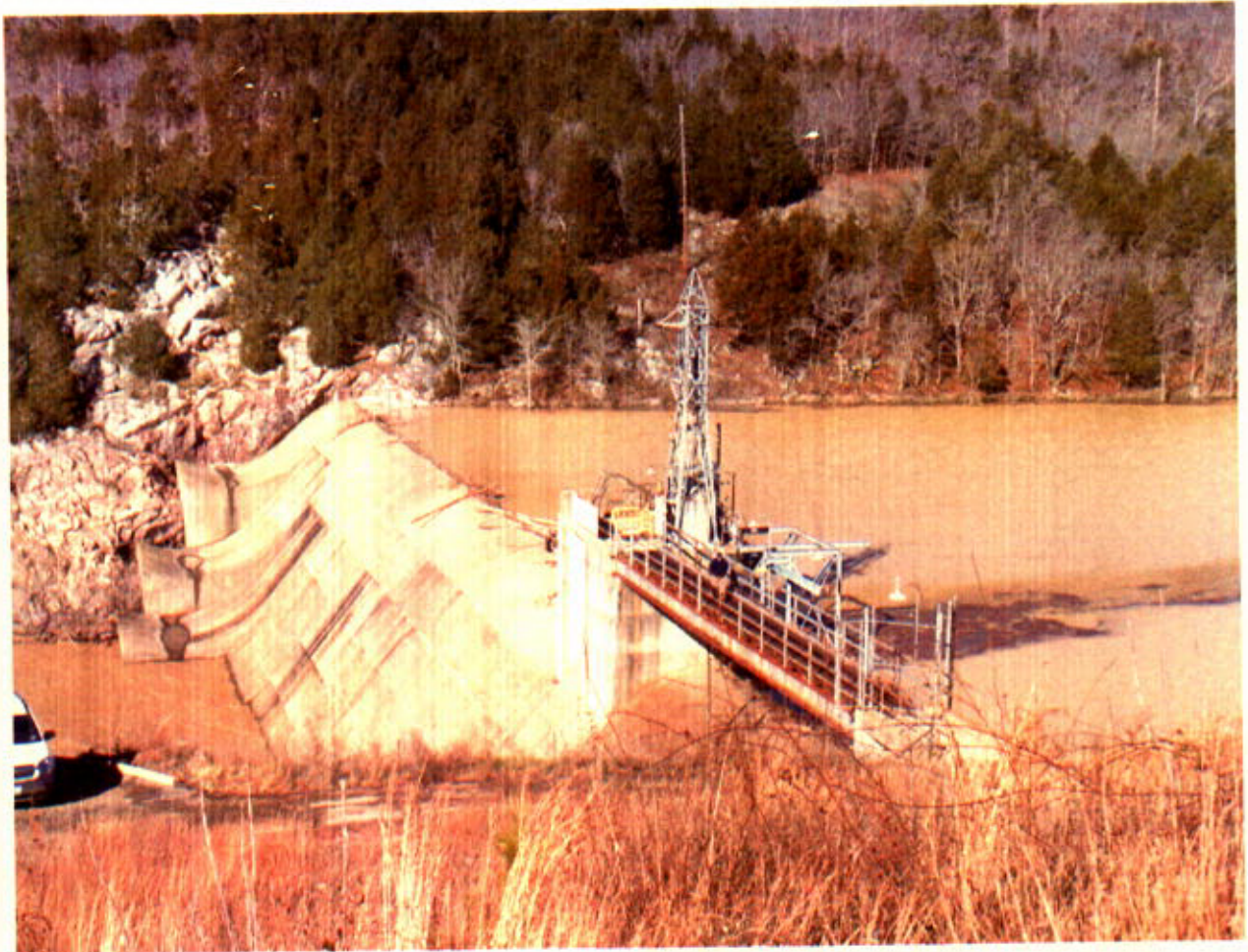
The photograph above shows the lower run of river dam the day after failure of the upper reservoir.
