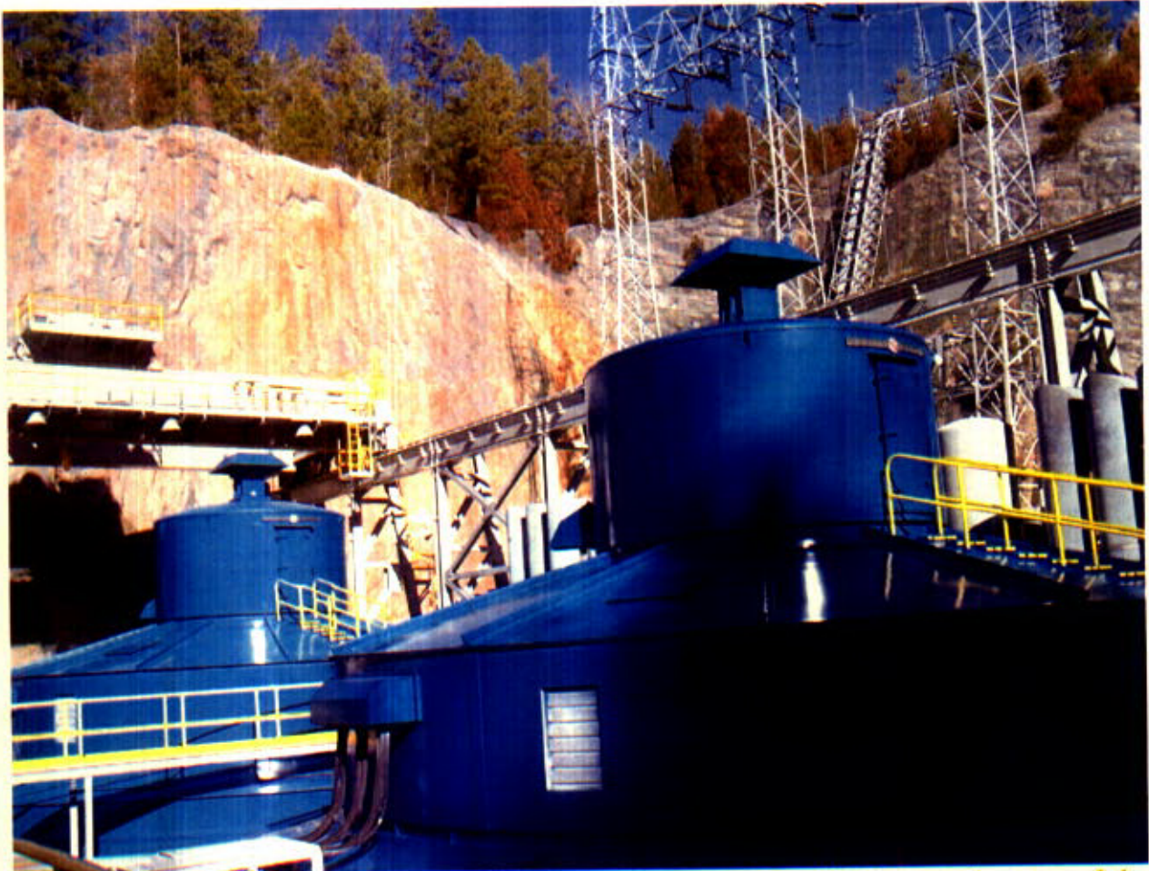
The above photograph is of the power site and the blue cylinders are the tops of the pumps/generators.
